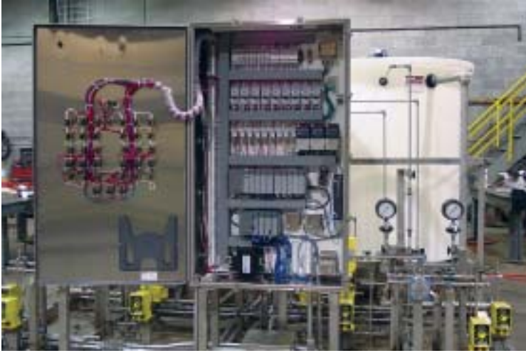
Electrical Control Panel
