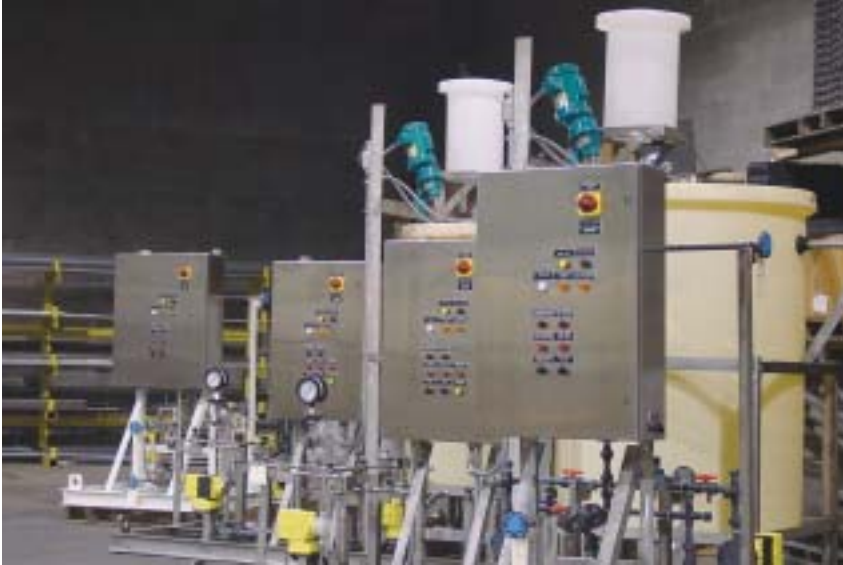
Chemical Feed Skids with Electrical Control Panels
