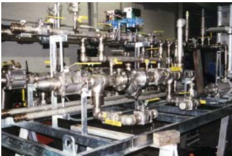
Ammonia Forwarding Skid
