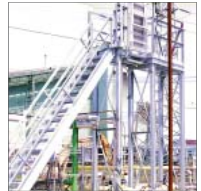
Aqueous Ammonia Unloading Platform
